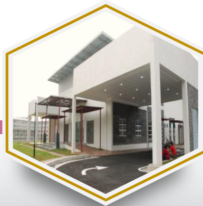
Engineering and Architecture Library Tel : 03-9769 2305
